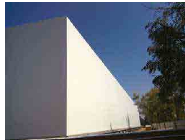
USED IN COMPOUND WALL
